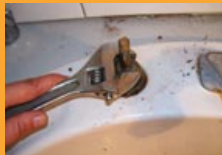
E. Unscrewing the tap body
