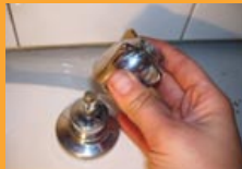
C. Pulling off the bit which turns
